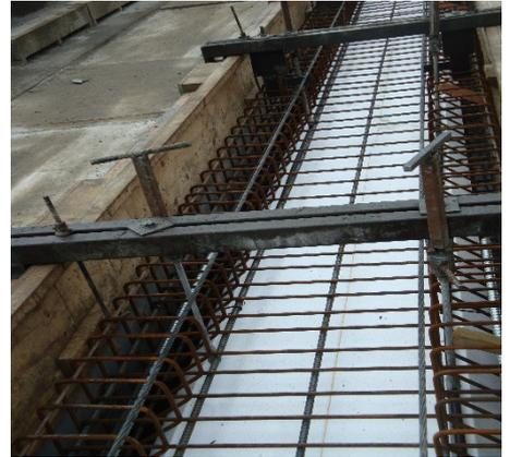
A typical mould loaded with reinforcing and prestressed cables ready to pour
